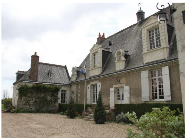
Figure 193 La façade Nord.
